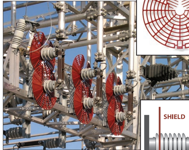
Model W-002R Mounted on 3 Hookstick Switches.
