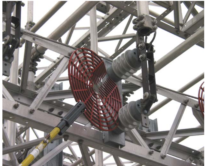
Figure 9: Install with Smooth & Steady Push
